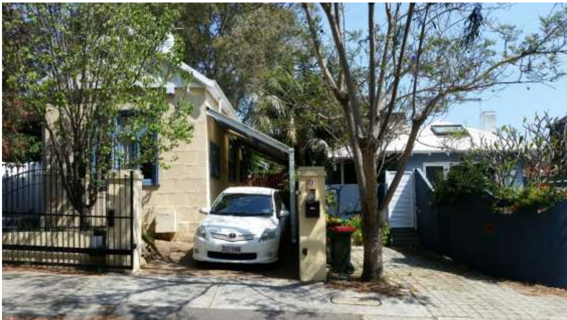
View of existing covered carport at 3 Wentworth Street
