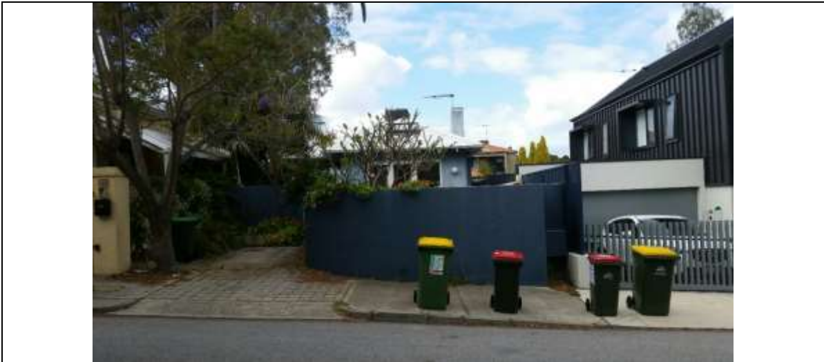
Front view of 1 Wentworth Street showing slope of lot
