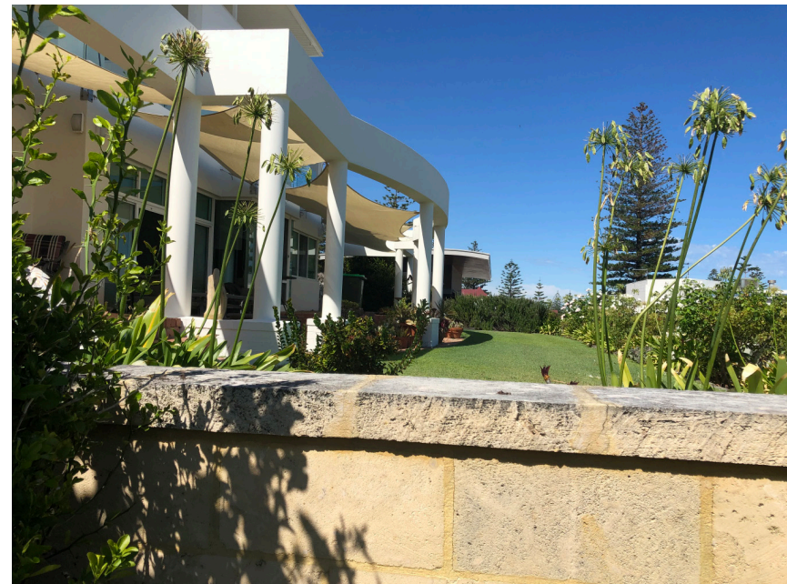
Figure 5: Looking south over boundary wall.
