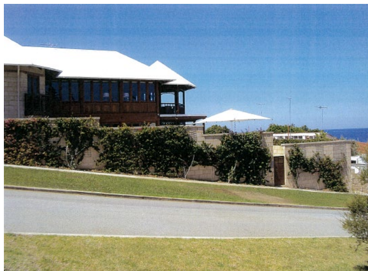
Above: Existing dwelling and retaining walls viewed from Princes Street
