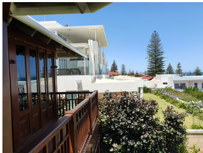
Above: Extent of existing overlooking over southern properties from 7 Avonmore Tce
