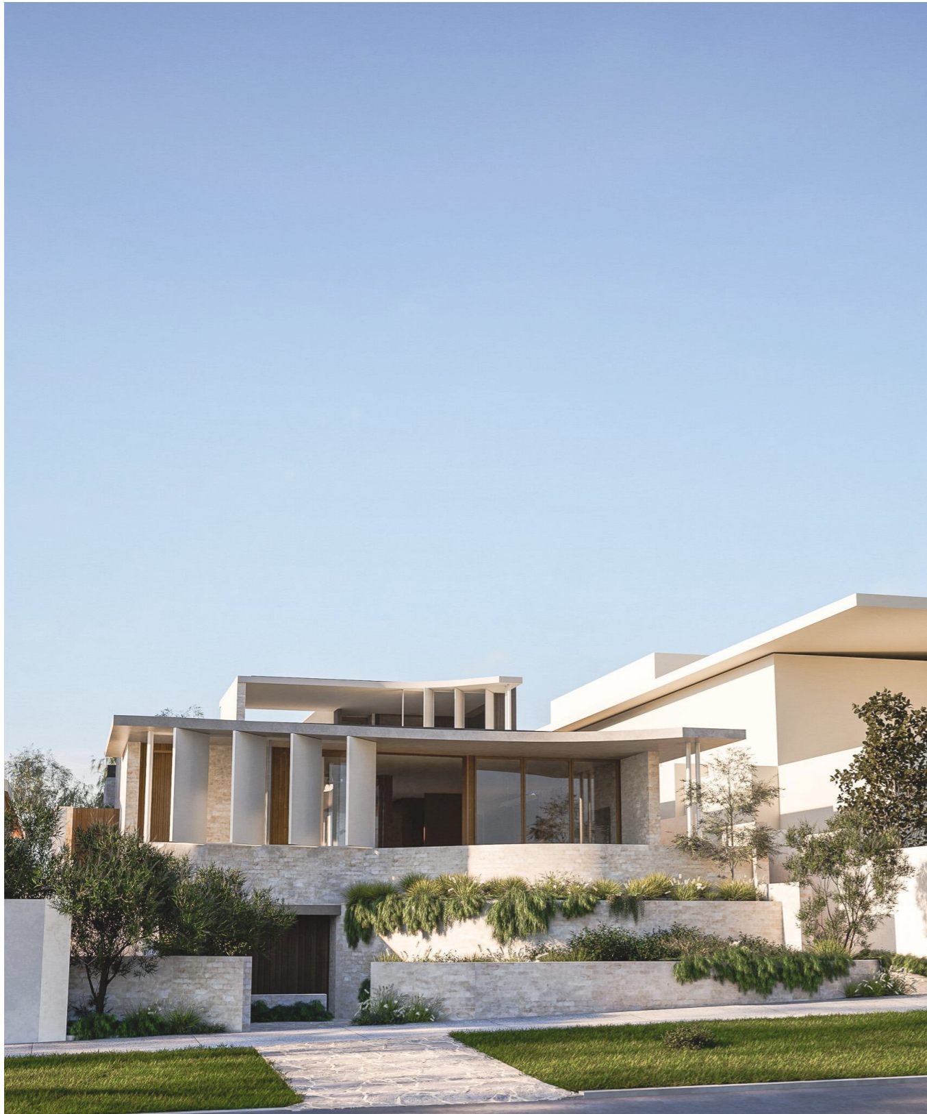
Ozone Parade streetscape. Facing south east
