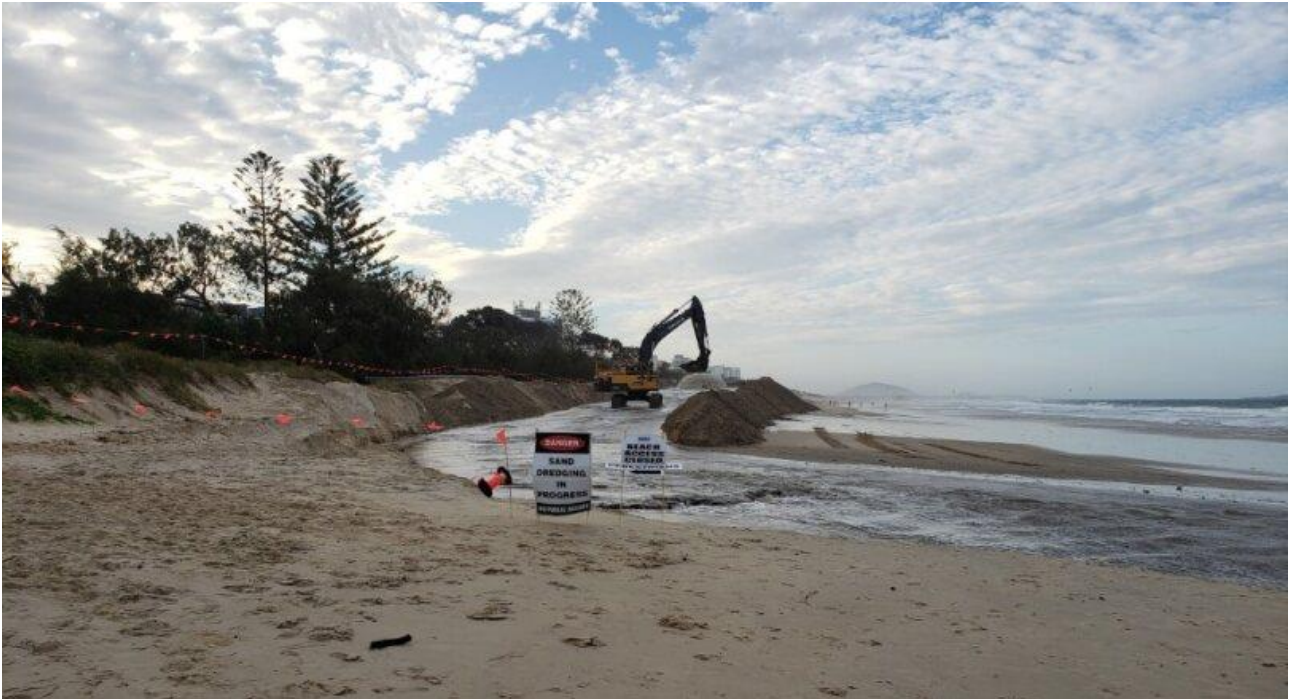
Figure 7-1 Beach nourishment underway at Sunshine Coast, QLD
