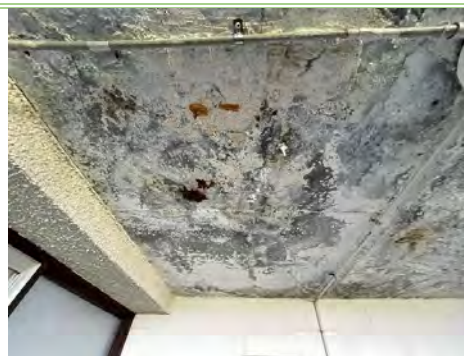
Figure 9: Drummy concrete and corrosion mark
