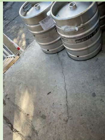
Figure 19: Crack evident on docking slab
