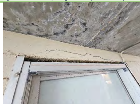
Figure 12: Beam cracks above door
