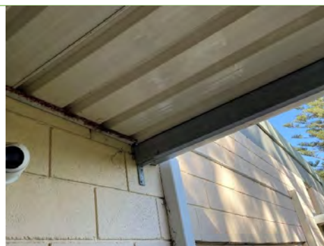
Figure 39: Surface corrosion on the canopy structure
