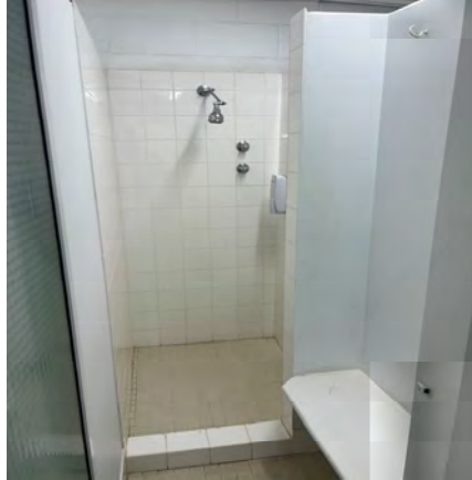
Typical shower cubical - showing hot and cold water taps and shower hose
