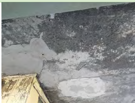
Figure 2: Drummy slab soffit
