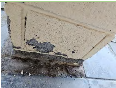
Figure 22: Deteriorating surface on concrete block columns.
