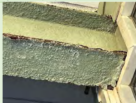
Figure 35: Steel beam on West Elevation - Severe corrosion
