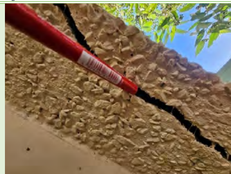
Figure 31: Windowsill panel crack width approx. 6mm
