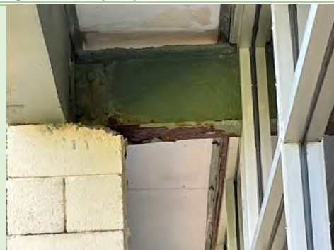
Figure 34: Steel beam on West Elevation - Severe corrosion
