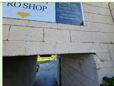
Figure 11: Concrete spalling on beam (external face)
