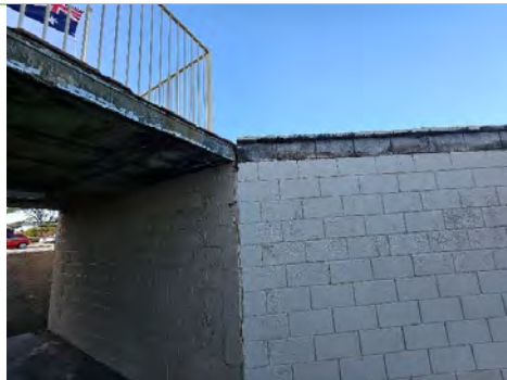
Figure 44: Crack at the joint
