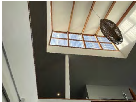
Figure 42: Roof Skylight Timber Frames
