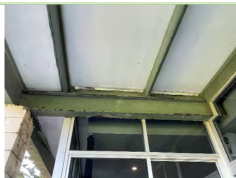
Figure 32: Balcony 1 exposed steel beam - Severe corrosion
