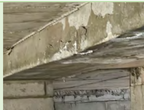
Figure 5: Close-up view of spalled concrete beam
