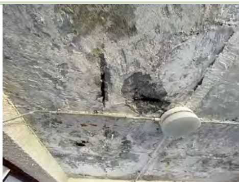
Figure 8: Corroded reinforcement on slab soffit
