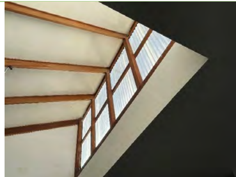
Figure 43: Roof Skylight Timber Frames
