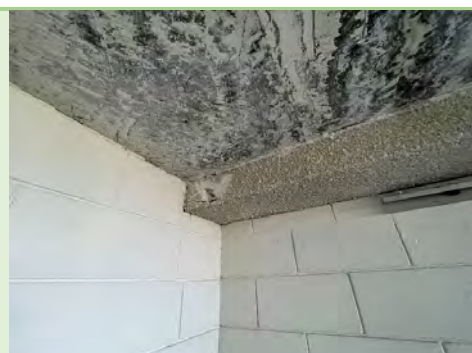
Figure 10: Concrete spalling on beam (Internal Face)
