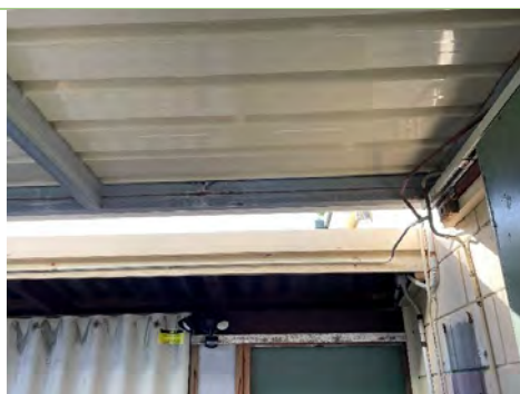
Figure 38: Surface corrosion on the canopy structure
