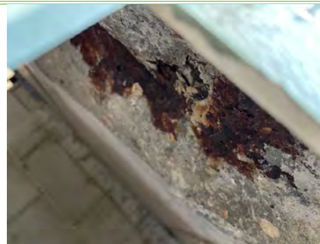
Figure 17: Slab soffit showing sign of corroded reinforcement
