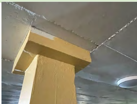
Figure 20: Internal concrete column in good condition.
