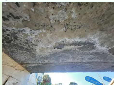
Figure 14: Drummy concrete to the slab soffit
