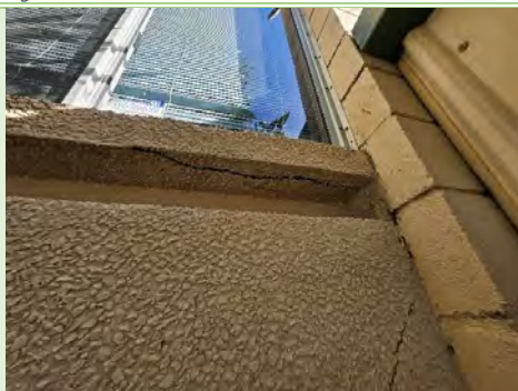
Figure 30: Major cracks on windowsill panel
