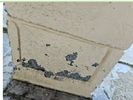
Figure 23: Deteriorating surface on concrete block columns
