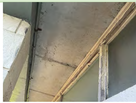
Figure 3: Drummy slab soffit
