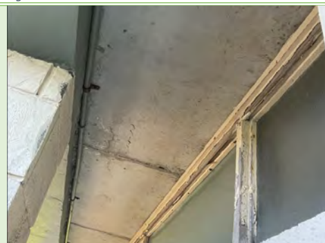
Figure 15: Drummy concrete to the slab soffit
