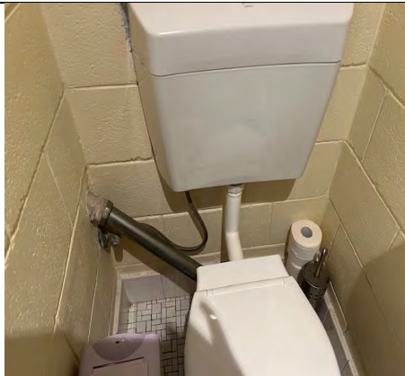
Toilet with exposed vent and water services
