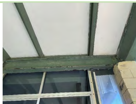
Figure 33: Balcony 2 exposed steel beam - Severe corrosion
