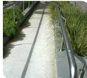
SS Handrail fixed to wall
