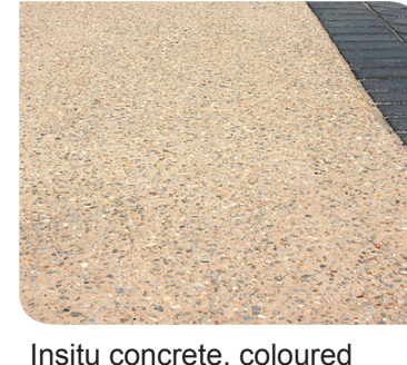
Insitu concrete, coloured exposed aggregate
