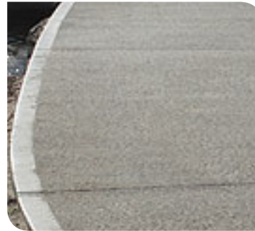
Insitu concrete, broom finish
