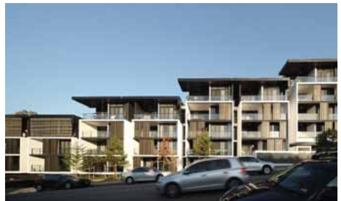
Development responds to the topography of the site
