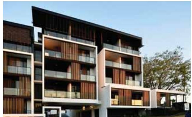
Example of access to parking area with minimal impact on public realm
