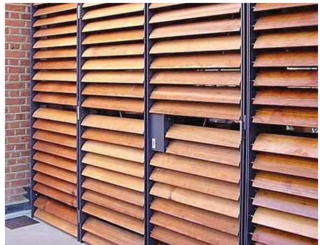
Plant louvre screening
