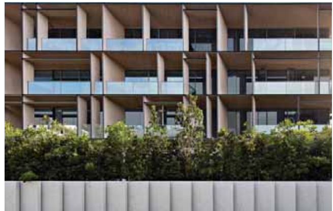
Balcony structures can be utilised to support activation of Marine Parade
