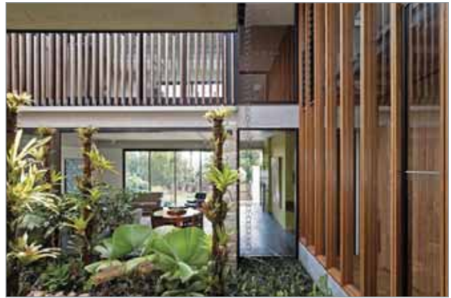
Built form to respond to amenity of the site and enhance residents experience
