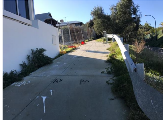
Figure 4 – Photo of existing constructed driveway to subject site
