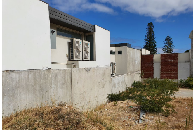
Above: View of existing walls without major openings on adjoining western lots
