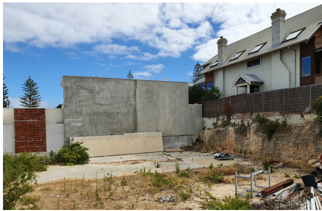
Above: View of existing wall without major openings on adjoining northern lot
