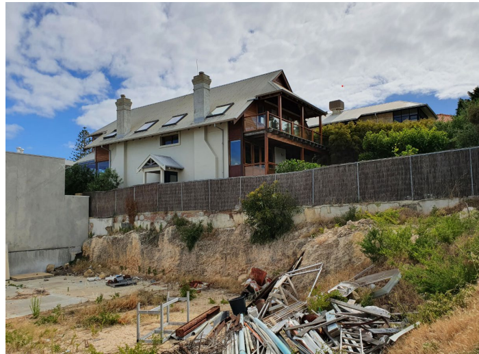
Above: Photo of existing excavation along eastern boundary
