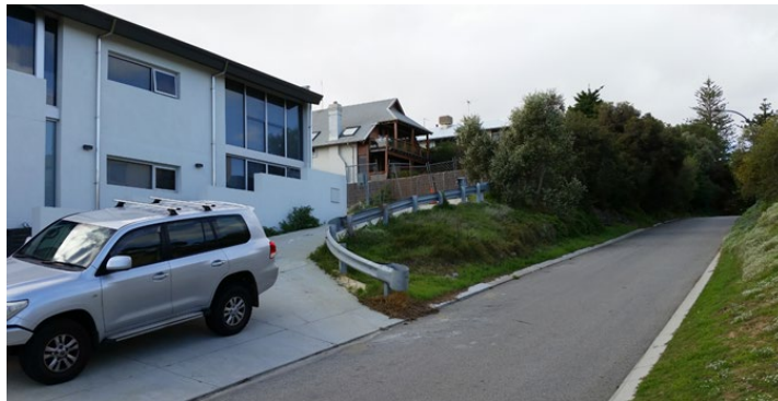
Above: Original crossover to Lots 505 & 506 following construction by the Town
