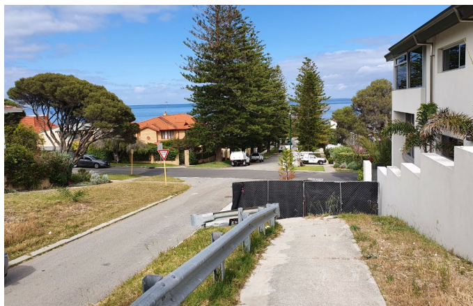
Above: Existing non-functional crossover and footpath looking west from Lot 506
