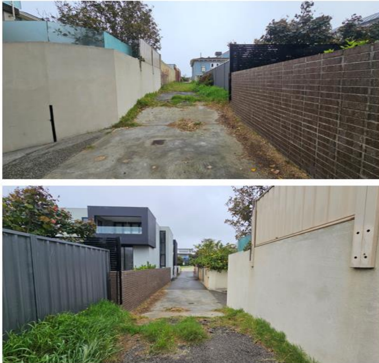
Figure 4: Photos showing difference in level
