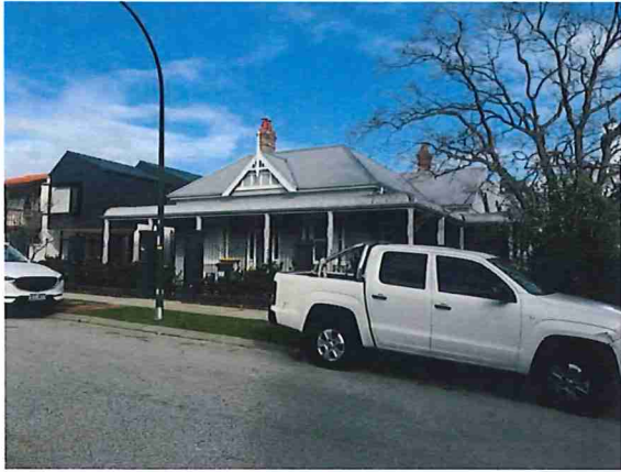
No 19 Perth Street: Front view looking southeast.
