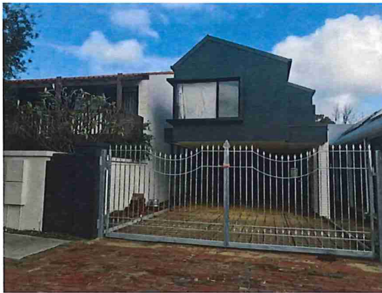
View showing the 2020 granny flat at No.19, on the east side of the residence.
