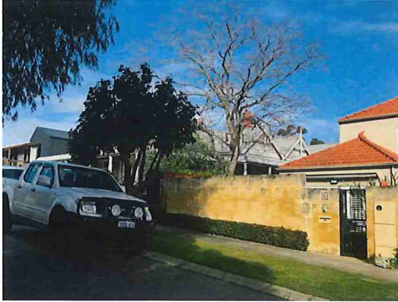
Perth Street streetscape south side: looking southeast showing (L-R) the 2020 No.19 granny flat, No.19 west gables, and No.15's stone fence and tiled roofs.
