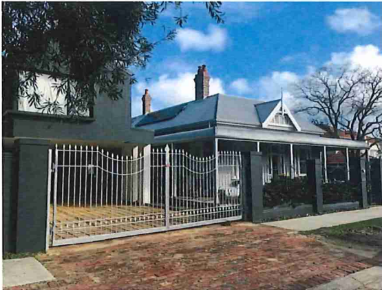
Perth Street streetscape south side: looking southwest showing No 19 residence and the 2020 granny flat (left).
