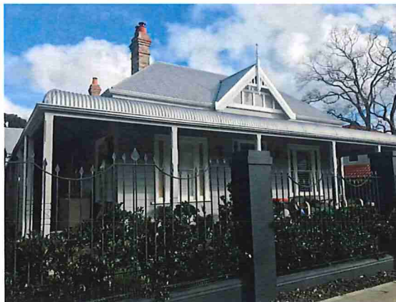
Front view of No.19 Perth Street.
