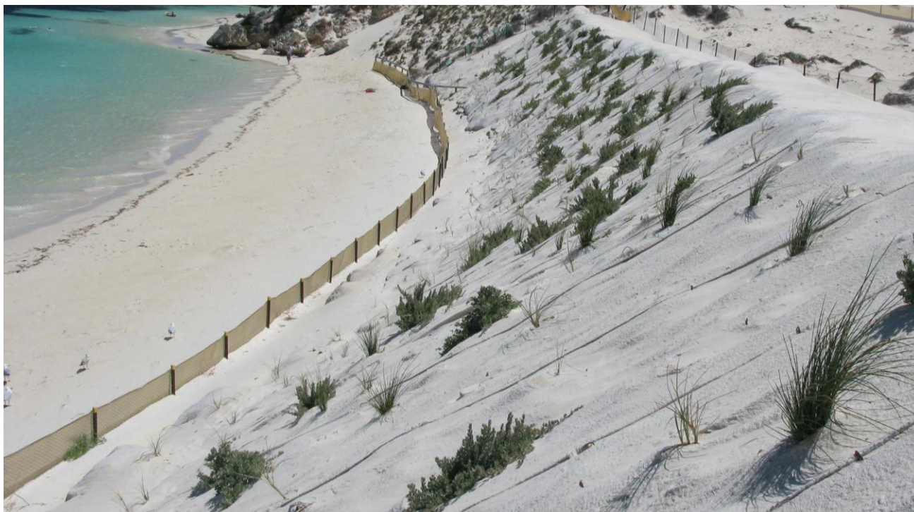
Figure 2: Example Jute matting on steep coastal dunes on Rottneest Island
