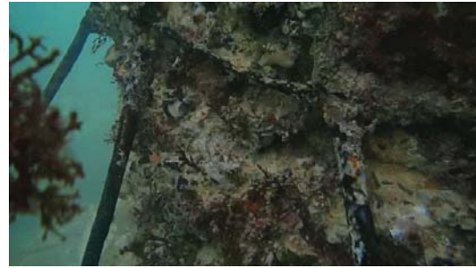
Figure 2-16 Part of ring visible at top of taper
