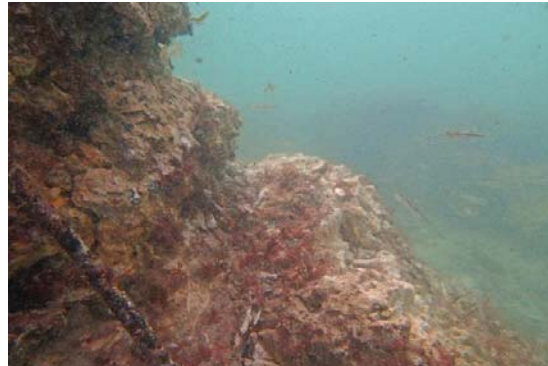
Figure 2-48 Uneven nature of foundations North-Eastern side
