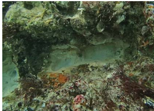
Figure 2-44 Soft clay-like material through rebar tapered section
