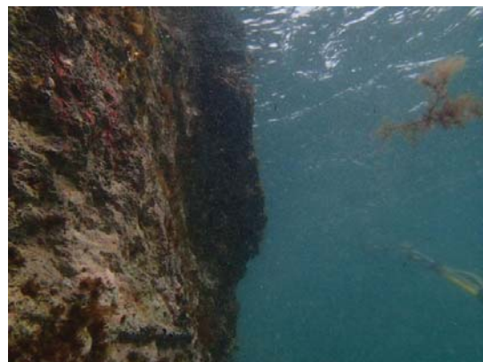
Figure 2-36 Pylon below scalloping at waterline
