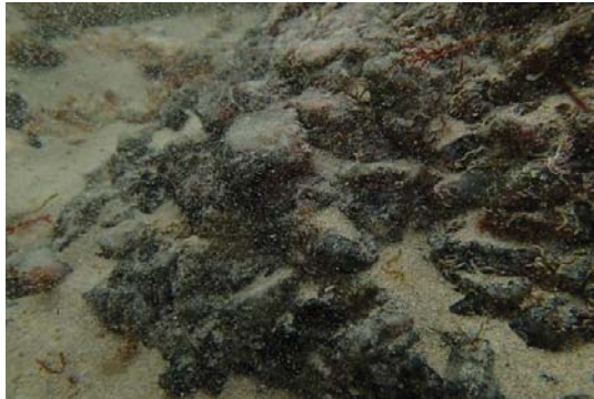
Figure 2-27 Bound blue metal South-Western side
