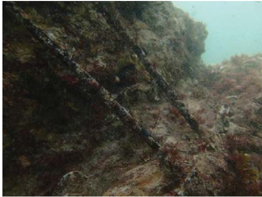
Figure 2-7 Rebar through top of tapered section
