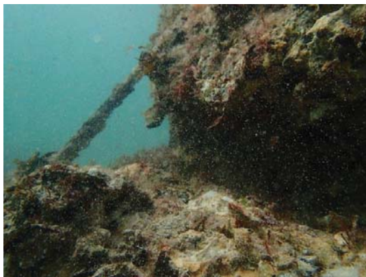
Figure 2-9 Rebar through top of tapered section
