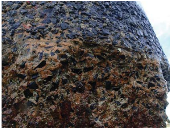
Figure 2-3 Concrete loss at waterline
