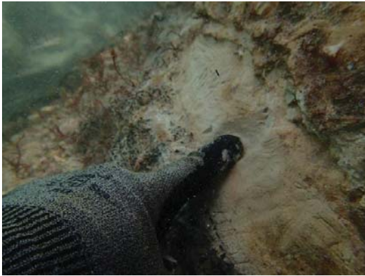
Figure 2-41 Soft clay-like material above blue metal section
