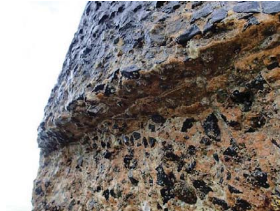
Figure 2-38 Cream mortar with blue metal aggregate above waterline
