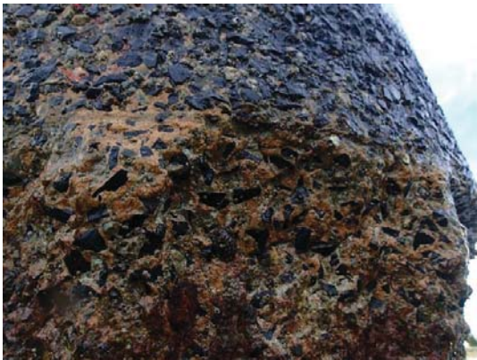
Figure 2-39 Exposed blue metal aggregate above waterline
