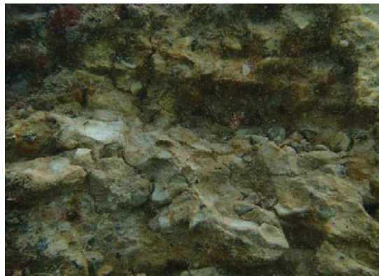
Figure 2-30 Cream mortar large stones showing cracking South-Eastern side
