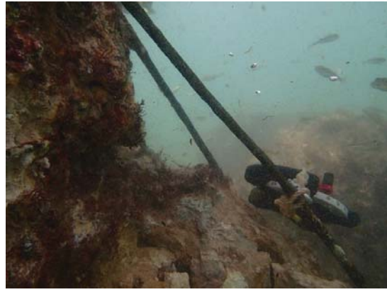
Figure 2-6 Rebar through top of tapered section
