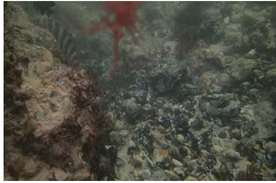
Figure 2-28 Loose blue metal Northern side
