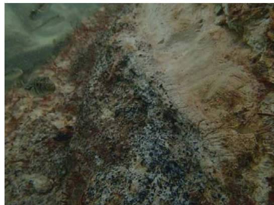
Figure 2-12 Soft concrete on lower taper
