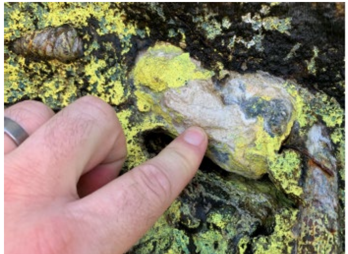
Figure 26: Possible evidence of embedded sacrificial anodes near exposed reinforcement.
