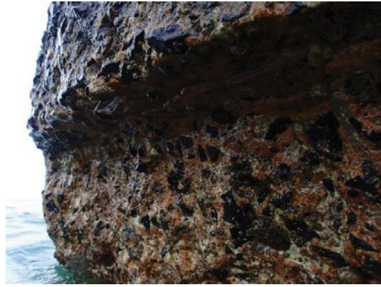
Figure 2-2 Concrete loss at waterline
