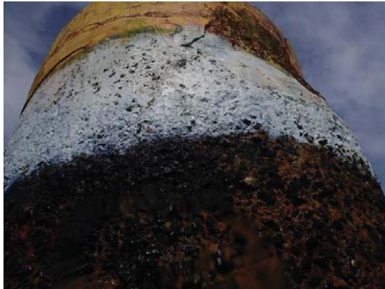
Figure 2-1 Pylon above waterline
