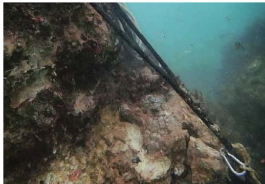
Figure 2-32 Cream mortar large stones degraded through rebar taper section
