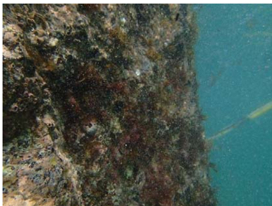
Figure 2-35 Pylon above rebar taper
