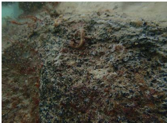
Figure 2-29 Cream mortar small stones South-Western side
