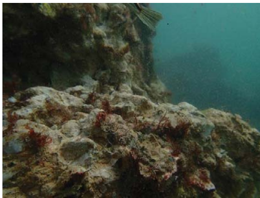
Figure 2-11 Crumbling concrete on taper
