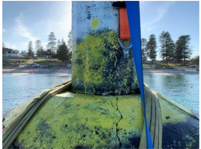
Figure 24: Upper section of the concrete pylon and bottom of the concrete mast
