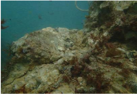
Figure 2-47 Uneven nature of foundations Eastern side
