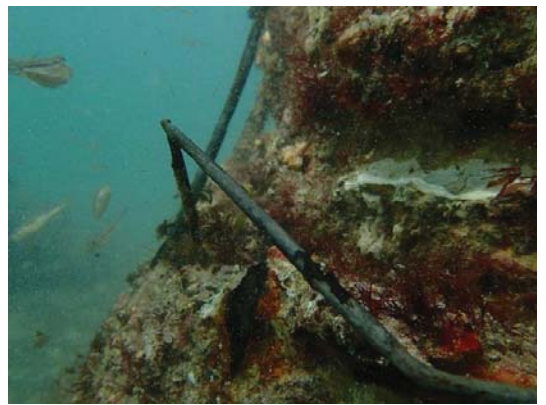
Figure 2-10 Rebar through top of tapered section
