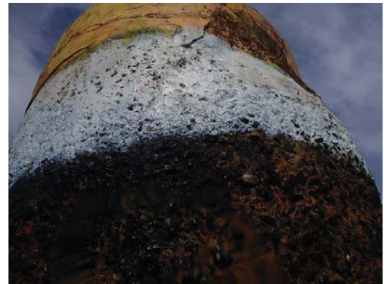
Figure 2-40 Pylon above waterline
