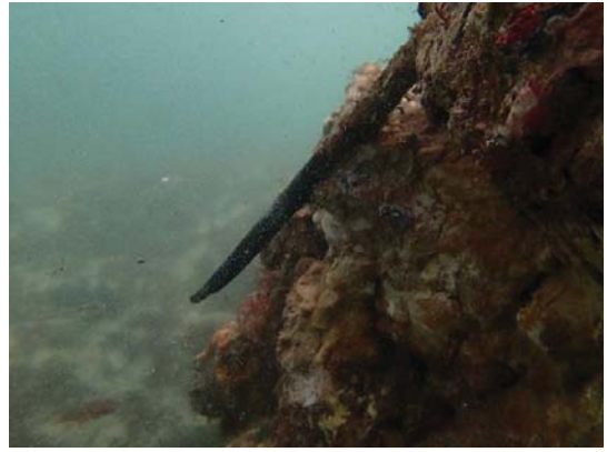
Figure 2-8 Rebar through top of tapered section
