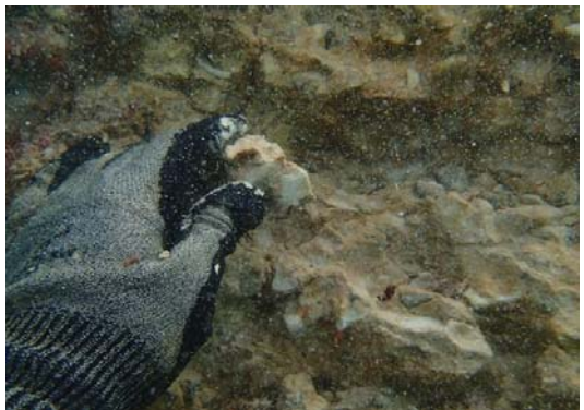
Figure 2-31 Cream mortar large stones diver removes aggregate by hand
