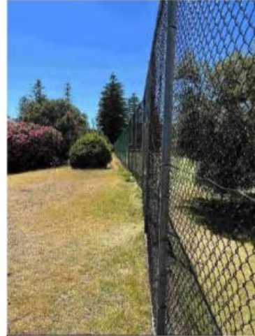
14 Northern boundary fence - Mid bend
