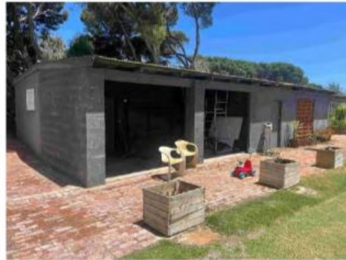
77 Old Curator's shed - East facade
