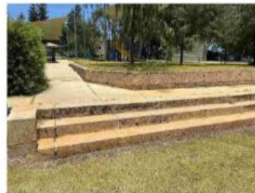
43 Internal concrete paths and stairs
