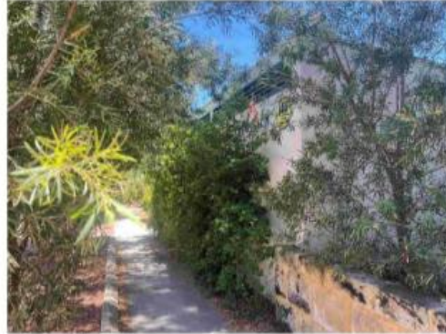
74 Curator's shed - South facade
