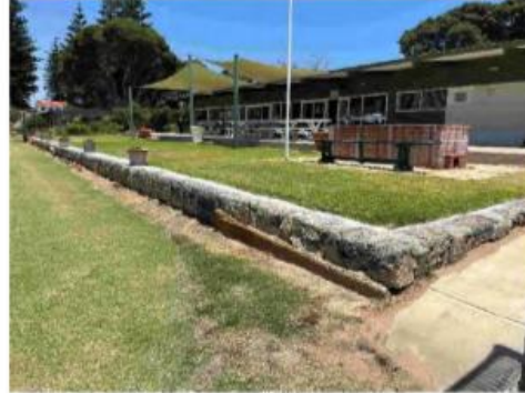
47 Minor internal retaining walls
