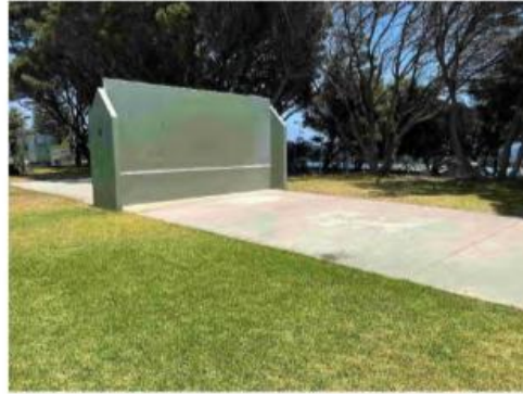
50 Concrete practice wall
