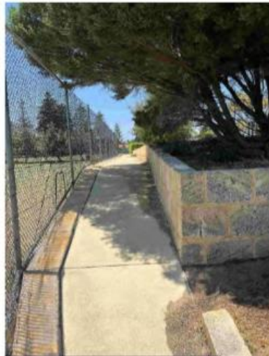
42 Internal concrete paths and stairs
