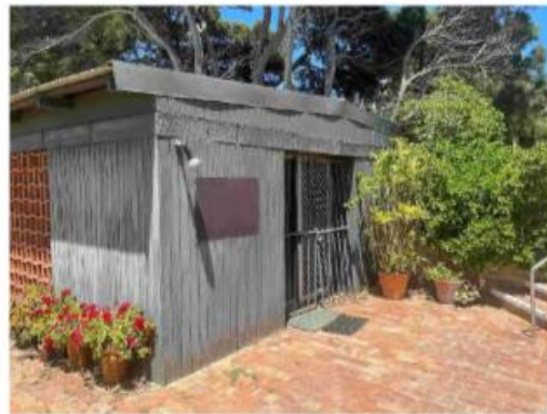
78 Old Curator's shed - North facade
