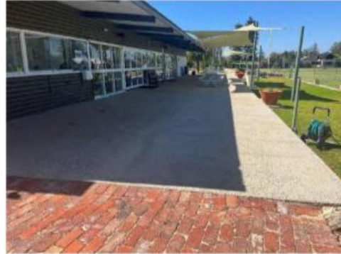
53 Exposed aggregate concrete veranda
