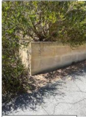
28 Southern boundary fence additional retaining terrace SW corner
