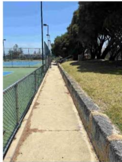
39 Internal concrete paths
