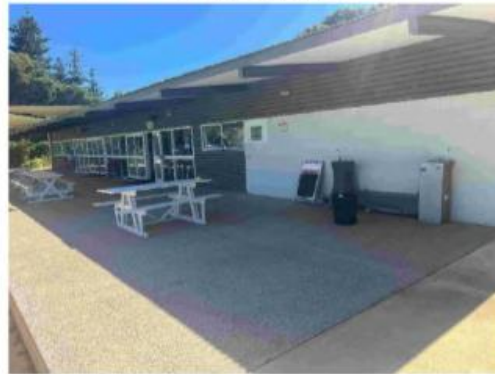
60 Main Building - East facade
