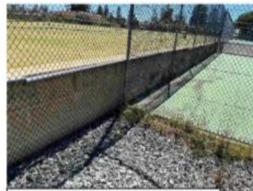
8 Western boundary fence - Hard court retaining north
