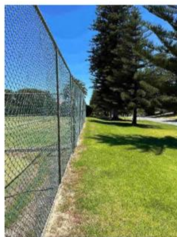
16 Eastern boundary fence - Minor rotation
