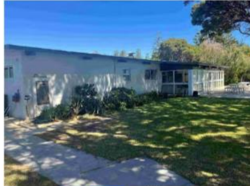
62 Main Building - West facade 1
