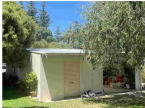
75 Curator's shed - Roof
