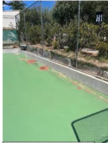
25 Southern boundary fence retaining wall
