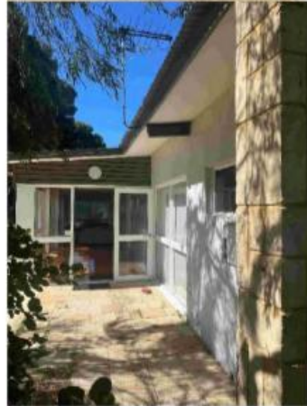
64 Main Building - West facade 3
