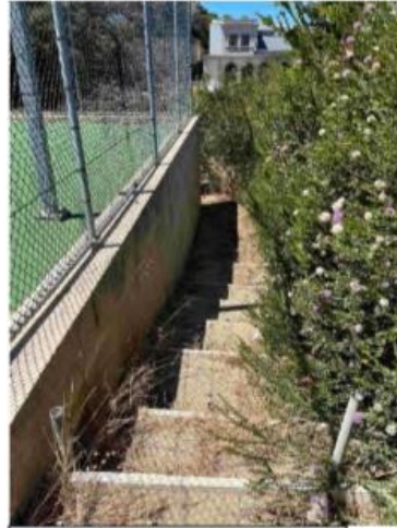
1 Retaining wall SW 1
