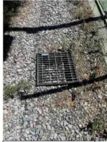
6 Western boundary fence - Drainage grate
