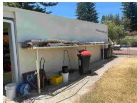
73 Curator's shed - West facade
