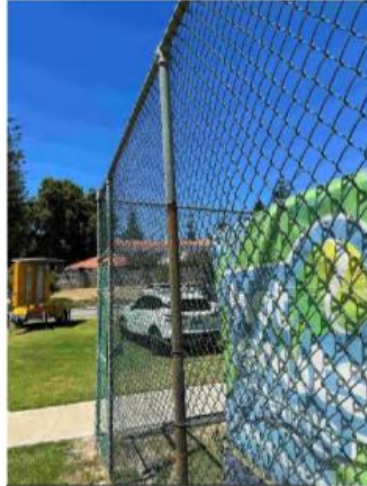
21 Eastern boundary fence - Minor rotation and rust
