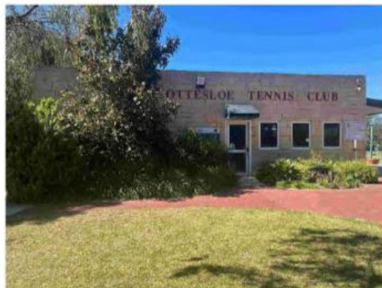
67 Main Building - South facade
