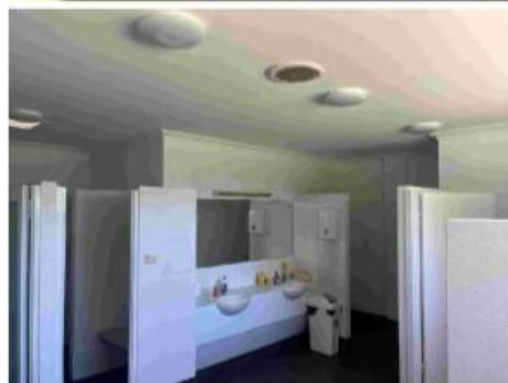
91 Main building - Mens Toilet
