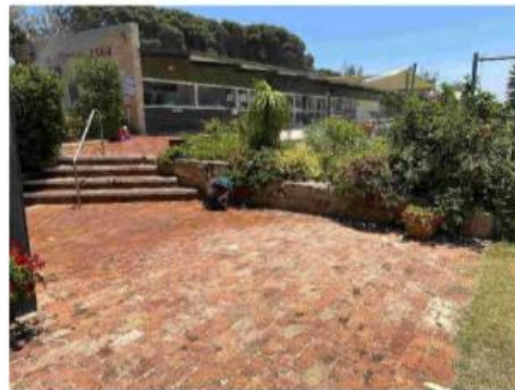
48 Minor internal retaining walls
