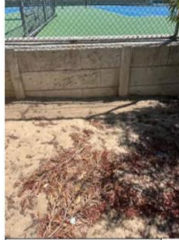
26 Southern boundary fence retaining wall
