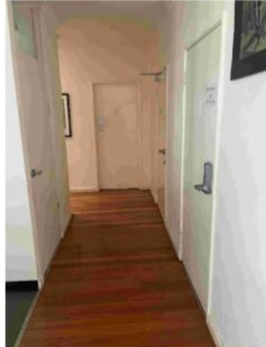
89 Main building - Toilet passage
