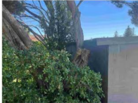
80 Old Curator's shed - West facade
