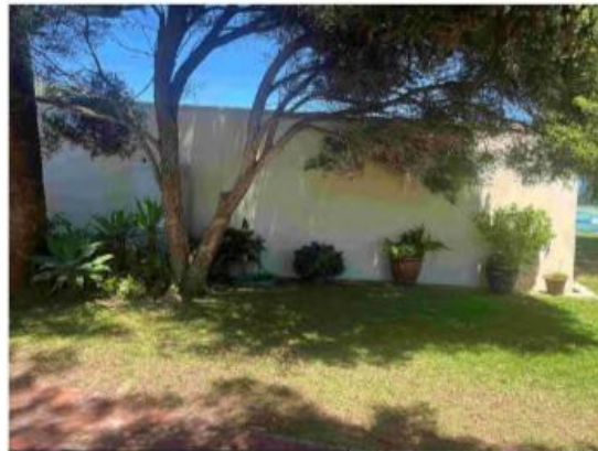
70 Curator's shed - East facade
