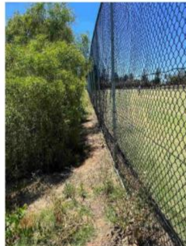
12 Northern boundary fence
