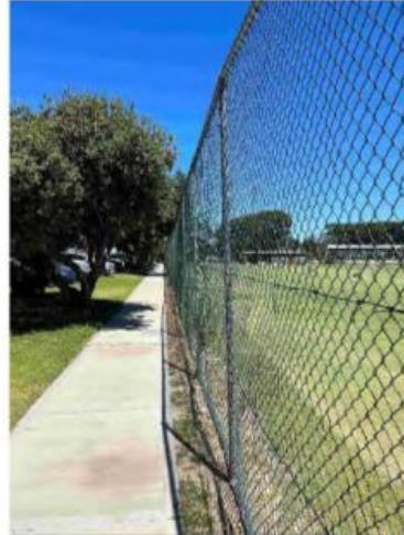
22 Southern boundary fence
