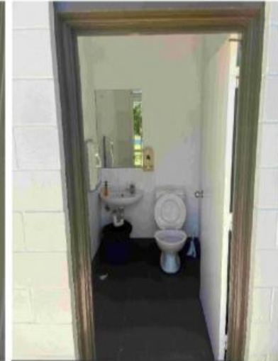
93 Main building - Public toilet
