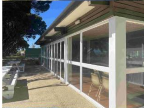
63 Main Building - West facade 2
