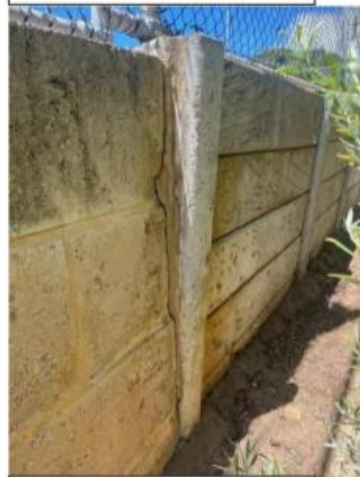
27 Southern boundary fence retaining change to limestone
