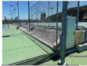
33 Hard court retaining 2
