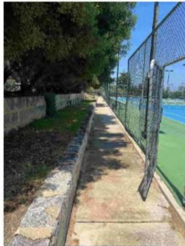
45 Minor internal retaining walls
