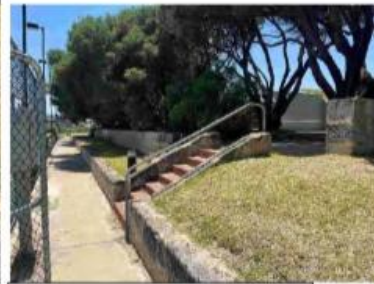
40 Internal concrete paths and stairs
