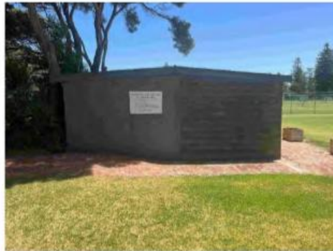
81 Old Curator's shed - South facade
