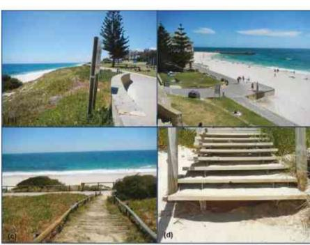
Figure 3-3 Infrastructure at Cottesloe Beach (a) majority of infrastructure/public amenity atop primary dune system (b) sea wall/amphitheatre extended to beach face (c) beach access paths both paved (background) and wooden (foreground) (d) undercutting of sediment under staircase to beach
