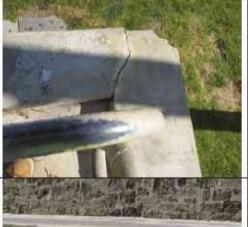
Typical Shrinkage crack on concrete retaining wall RW5
