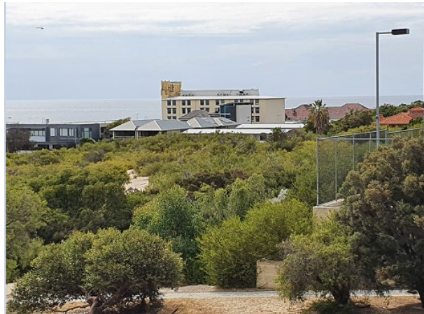
Above: View of existing OBH building taken from Cottesloe Civic Centre.
