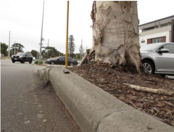
Figure 2: *Melaleuca quinquenervia* causing damage to road and curbing on Jarrad St.
