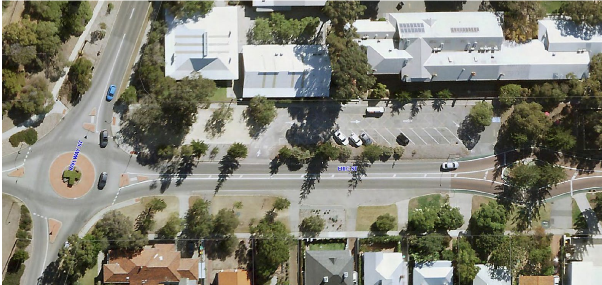
Fig 11: Existing Kiss and Drop parking facility.
