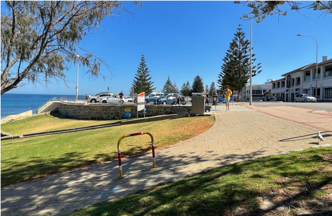
Photograph 7: The work begins at the access roadway dating from the inter-war period. The limestone walls, stairs, railings and car park will be removed in the renewal process and the land profile will more closely resemble that of the foreground. The Cottesloe Beach Hotel is to the right. Griffiths Architects January 2021.
