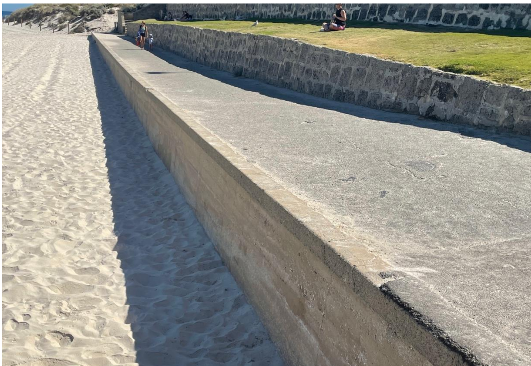
Photograph 10: The inter-war concrete sea wall remains in place. Griffiths Architects January 2021.
