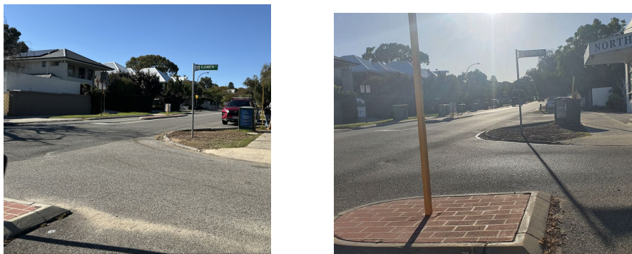
Figure 1: Obstructed line of sight when parking bays are occupied vs unobstructed line of sight
