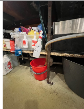
Coffee machines drain into the bucket
