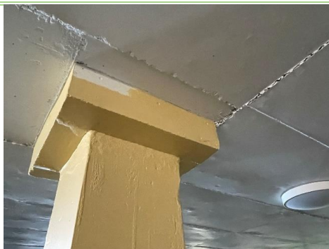
Figure 20: Internal concrete column in good condition.
