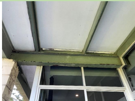
Figure 32: Balcony 1 exposed steel beam - Severe corrosion
