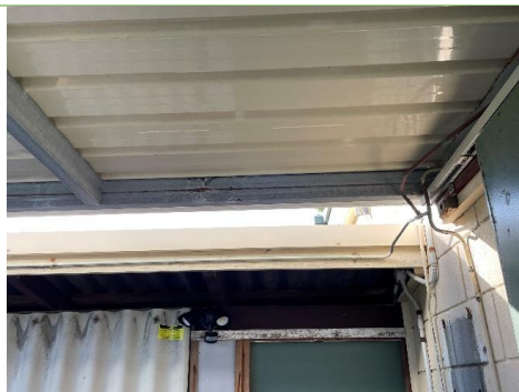
Figure 38: Surface corrosion on the canopy structure
