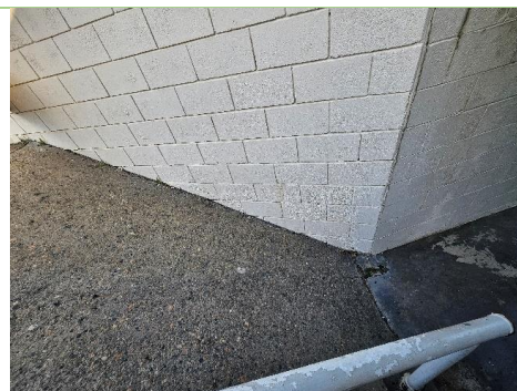
Figure 45: Crack at the joint
