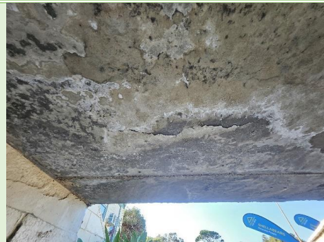
Figure 14: Drummy concrete to the slab soffit
