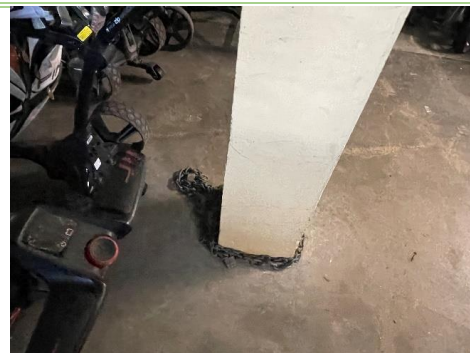
Figure 21: Internal concrete column in good condition.
