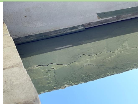
Figure 37: Concrete perimeter beam on North Elevation - Concrete Cracking
