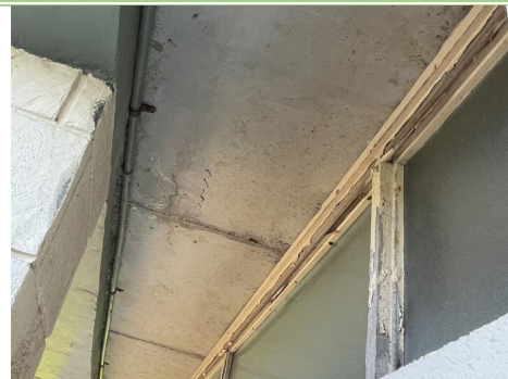
Figure 3: Drummy slab soffit
