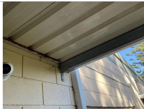
Figure 39: Surface corrosion on the canopy structure
