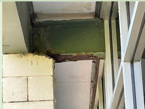
Figure 34: Steel beam on West Elevation - Severe corrosion
