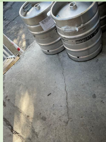
Figure 19: Crack evident on docking slab
