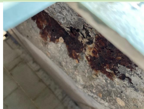
Figure 17: Slab soffit showing sign of corroded reinforcement
