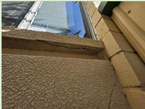
Figure 30: Major cracks on windowsill panel
