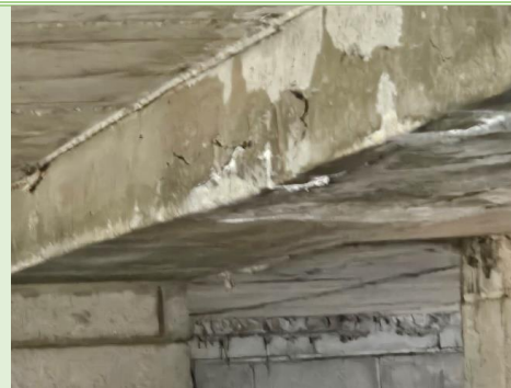
Figure 5: Close-up view of spalled concrete beam
