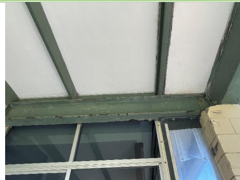
Figure 33: Balcony 2 exposed steel beam - Severe corrosion
