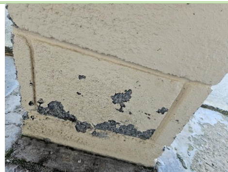
Figure 23: Deteriorating surface on concrete block columns
