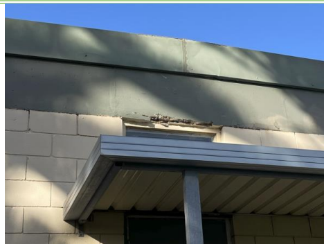
Figure 36: Concrete perimeter beam on North Elevation - Concrete spalling & corroded reinforcement
