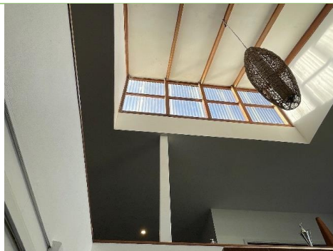
Figure 42: Roof Skylight Timber Frames
