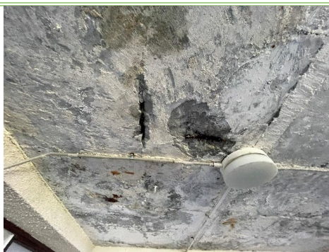
Figure 8: Corroded reinforcement on slab soffit
