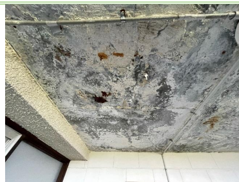
Figure 9: Drummy concrete and corrosion mark
