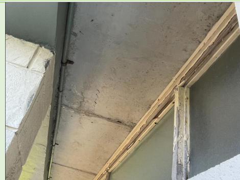
Figure 15: Drummy concrete to the slab soffit
