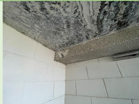
Figure 10: Concrete spalling on beam (Internal Face)
