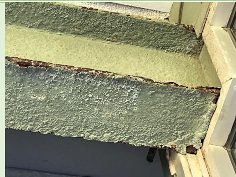
Figure 35: Steel beam on West Elevation - Severe corrosion
