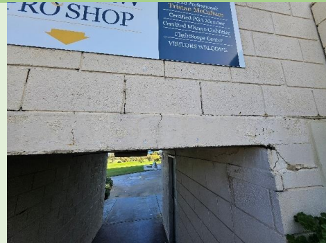
Figure 11: Concrete spalling on beam (external face)
