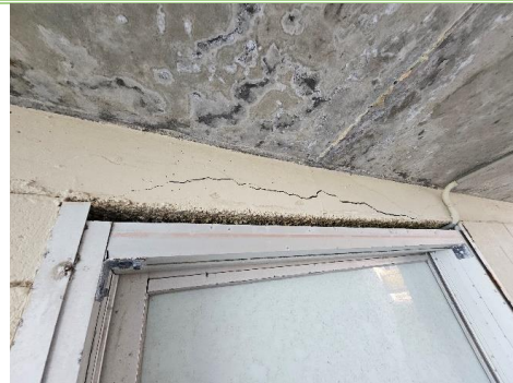
Figure 12: Beam cracks above door
