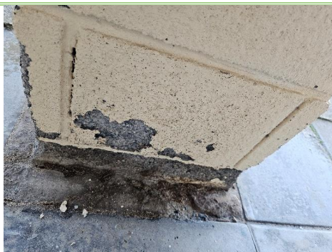
Figure 22: Deteriorating surface on concrete block columns.
