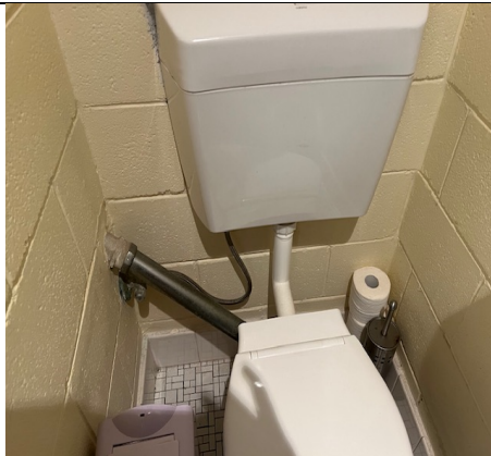
Toilet with exposed vent and water services
