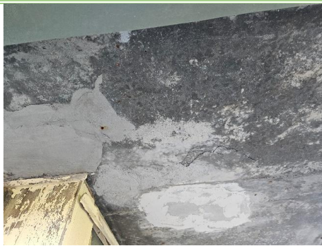
Figure 2: Drummy slab soffit
