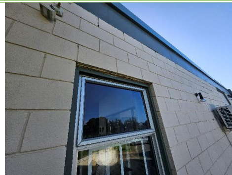
Figure 29: Lintel on South elevation - Moderate corrosion
