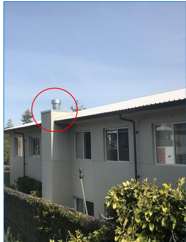
Figure 4 – Image looking south-west to eastern elevation of No. 24 Avonmore Terrace. The flue boxing demonstrating the approximate height of the proposed ground floor southern boundary wall on the subject site.
