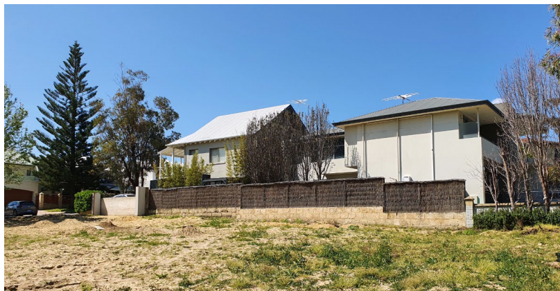
Above: View from site of adjoining eastern property (offices)
