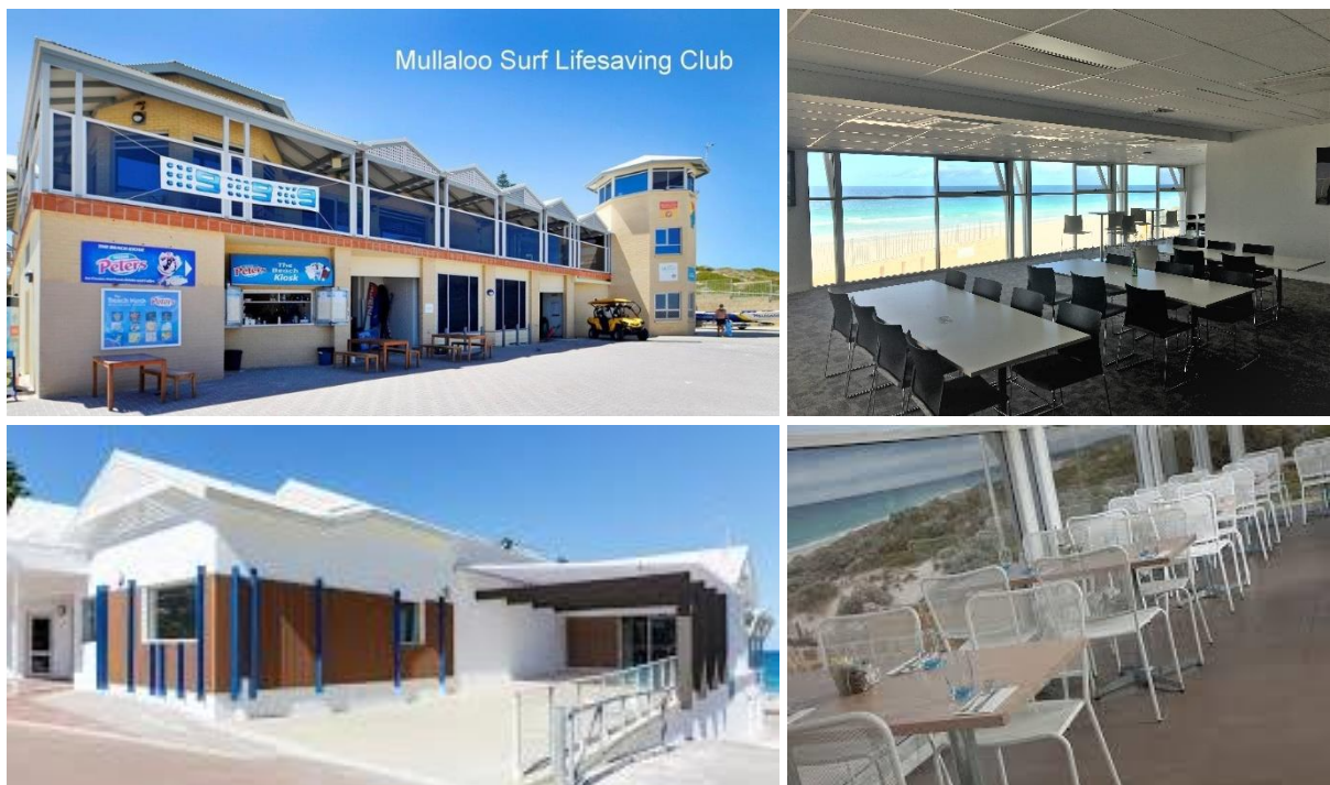
Upper left, clubrooms from the west; upper right members lounge; bottom left entry from carpark; bottom right new café seating (leased out)
