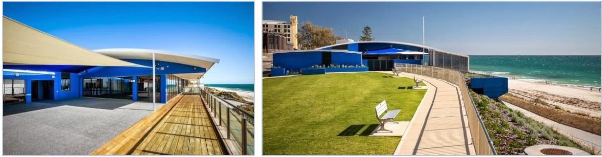
North Cottesloe upper deck and right, north elevation
