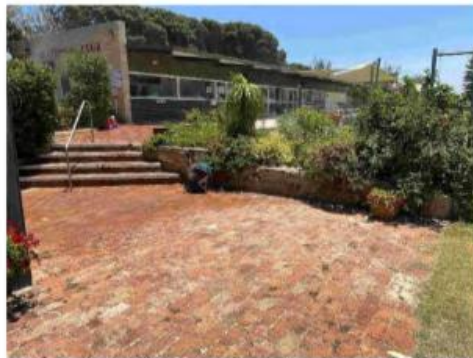
48 Minor internal retaining walls
