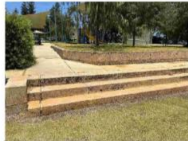
43 Internal concrete paths and stairs
