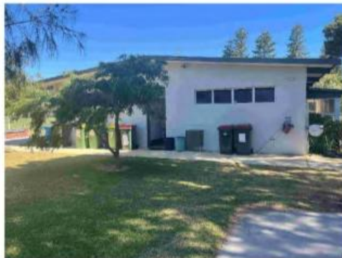
61 Main Building - North facade
