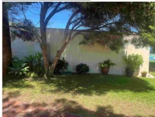
70 Curator's shed - East facade
