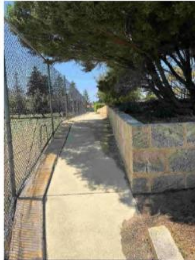
42 Internal concrete paths and stairs
