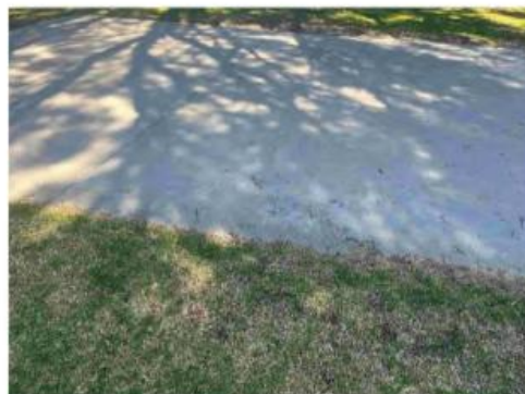
52 Concrete practice wall - Minor cracking
