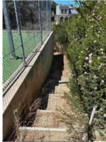
1 Retaining wall SW 1
