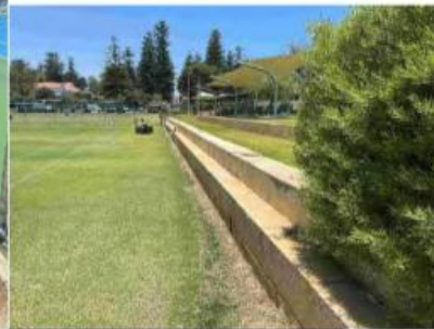
46 Minor internal retaining walls
