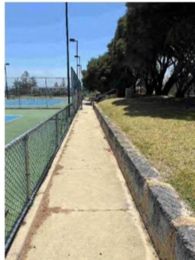
39 Internal concrete paths
