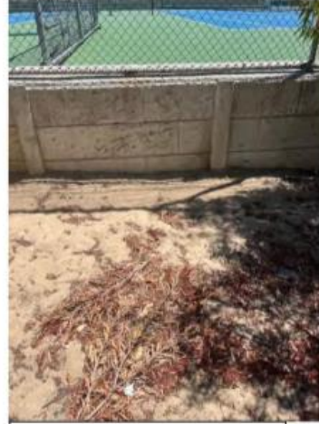
26 Southern boundary fence retaining wall
