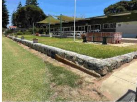
47 Minor internal retaining walls
