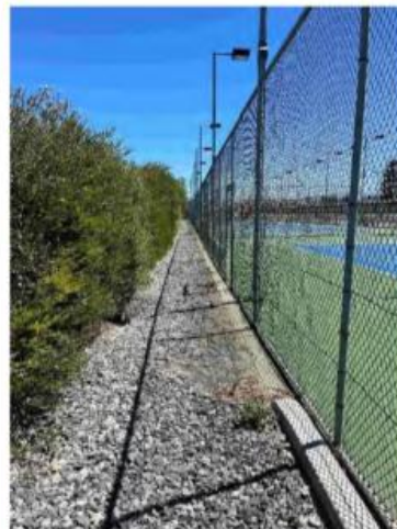
4 Western boundary fence
