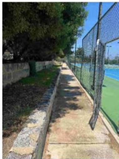
45 Minor internal retaining walls
