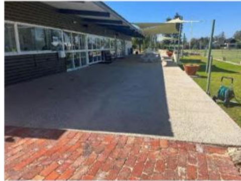
53 Exposed aggregate concrete veranda
