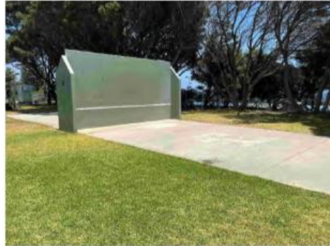
50 Concrete practice wall
