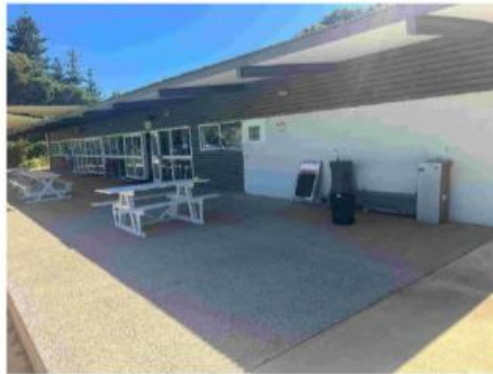
60 Main Building - East facade
