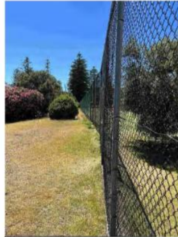
14 Northern boundary fence - Mid bend
