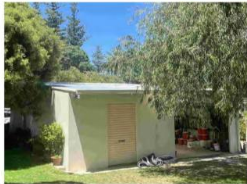
75 Curator's shed - Roof
