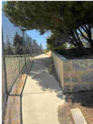
42 Internal concrete paths and stairs
