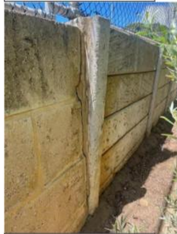
27 Southern boundary fence retaining change to limestone
