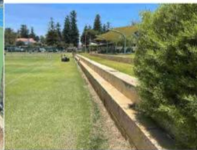
46 Minor internal retaining walls
