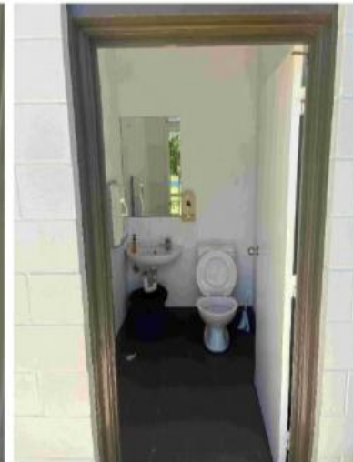
93 Main building - Public toilet
