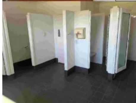
90 Main building - Ladies Toilet
