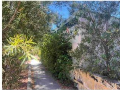
74 Curator's shed - South facade
