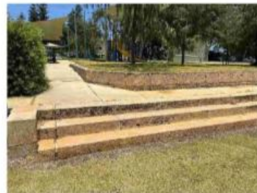
43 Internal concrete paths and stairs
