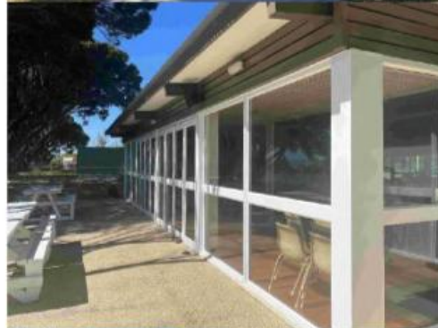
63 Main Building - West facade 2
