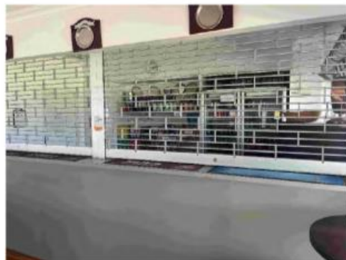
85 Main building - Bar area
