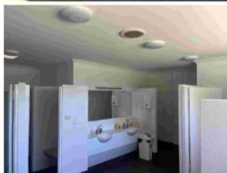
91 Main building - Mens Toilet
