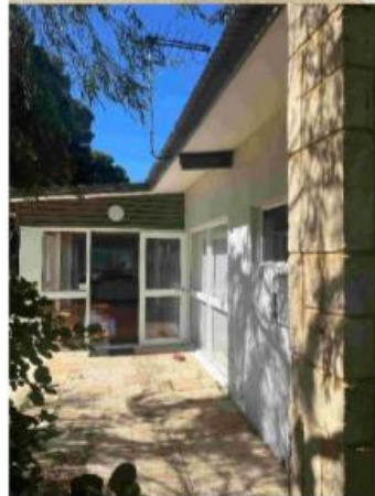
64 Main Building - West facade 3
