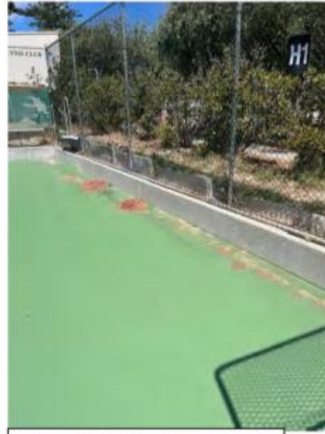
25 Southern boundary fence retaining wall
