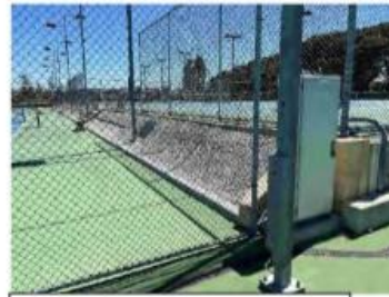
33 Hard court retaining 2
