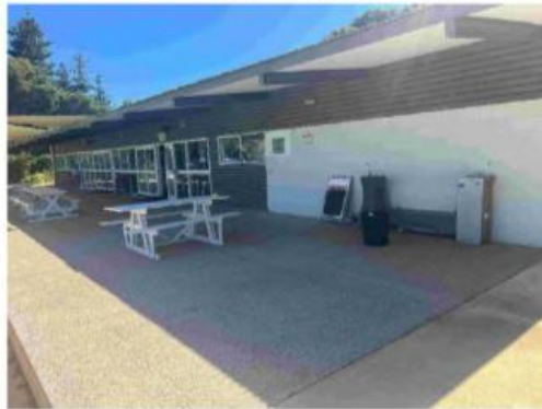
60 Main Building - East facade
