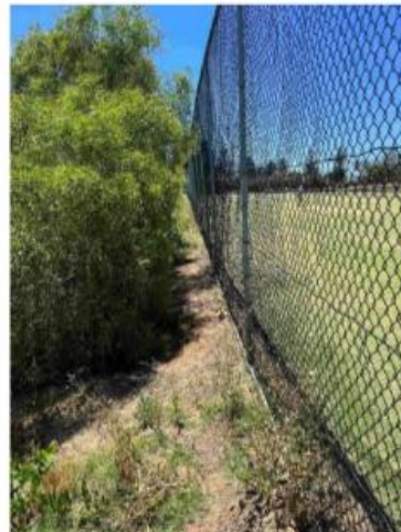
12 Northern boundary fence
