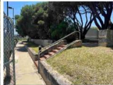
40 Internal concrete paths and stairs
