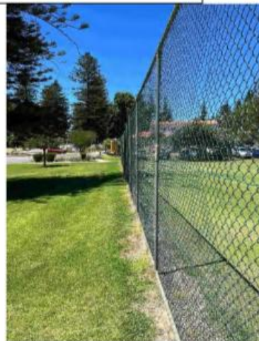
20 Eastern boundary fence - SE corner
