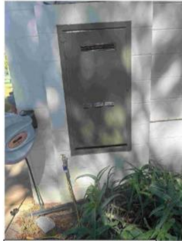
65 Main Building - West facade HWS
