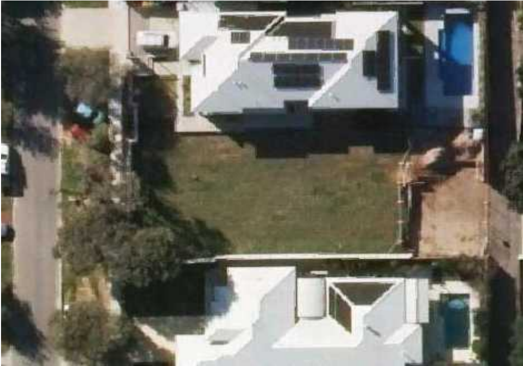
Above - Aerial photo (prior to construction)
