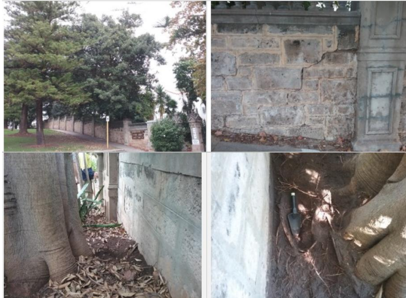
Figure 2: Tree roots damaging boundary wall
