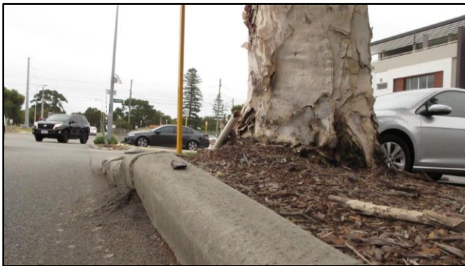
Figure 2: Melaleuca quinquenervia causing damage to road and curbing on Jarrad St.
