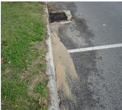
Sand drift into drains
