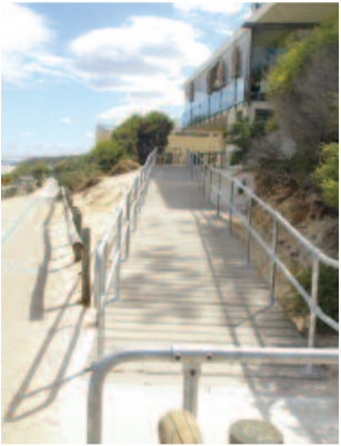
Recently installed ramp for access to North Cott toilets below Barchetta restaurant
