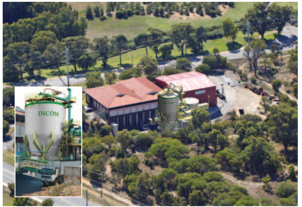
Aerial view of the Brockway site shows the new DiCOM installation, and inset, a close-up of the first digester vessel.
